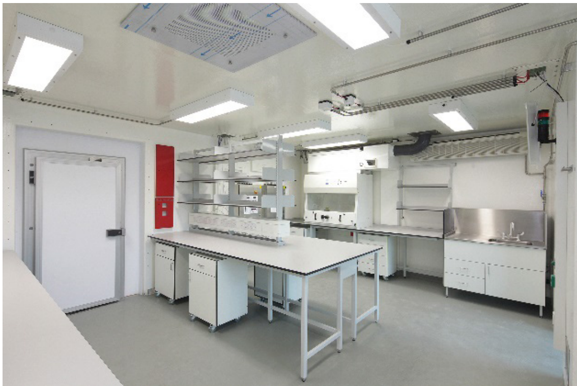
Copyright: Shepherd Construction.
